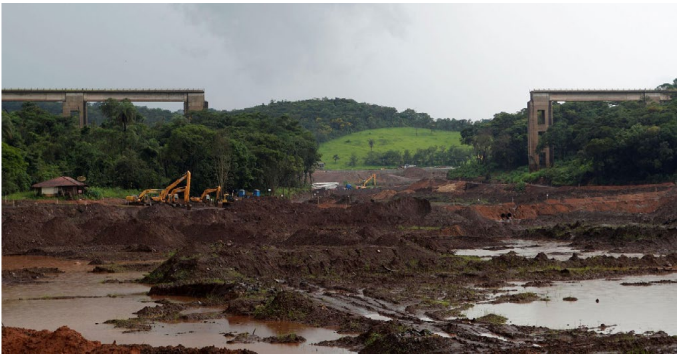
Vale's tailings dam in Brumadinho
